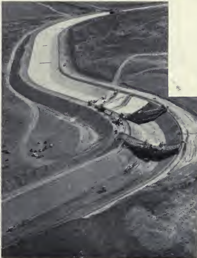
MACHINES THAT WALKED A MILE A WEEK. —At left, lining operations in the Moin Conol. In the background is the fork where the East Low and West Conols take off from the Moin Conol. Below, the West Conol. Both photos by H. E. Foss, Region 1 photographer.
